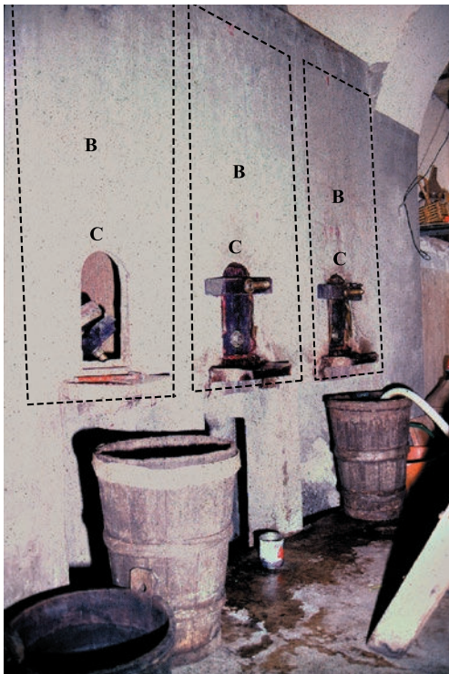
Fig. 42. Fermentation vats in a domestic winepress in Monte-Laterone, Tuscany, Italy: B–vats, C–vats’ openings (photography: Y. Dray).
